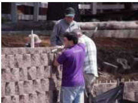
Jim Keene supervises construction of the new waterfront.
